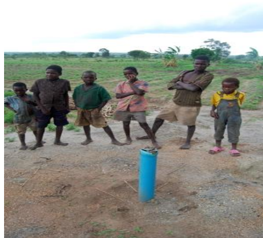
Borehole Drilled, awaiting pump
