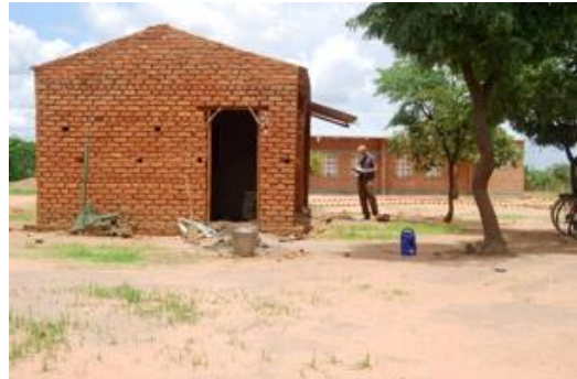
Chicken khola, under construction.
