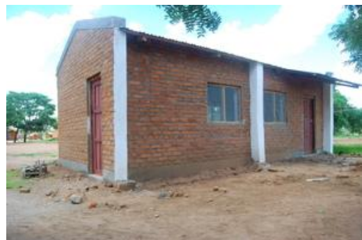
Chicken Khola building, finished.
